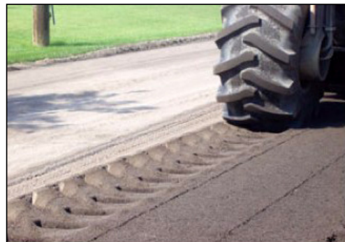
Material before mixing (left) and after mixing (right). Note the fly ash on the left side.
