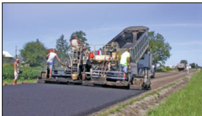
Asphalt placed over treated pavement base materials
