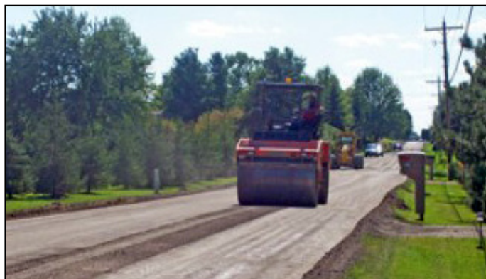
Compaction of the FDR base layer in Delaware County
