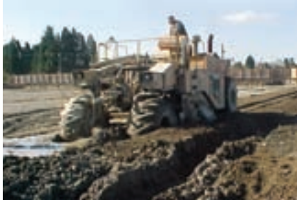
Incorporation of Class C fly ash into wet soil to facilitate moisture reduction.
