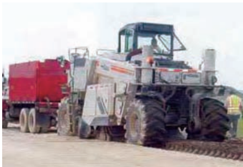
USH near Fort Atkinson, Wisconsin: Subgrade being mixed with fly ash placed over it (the red tanker provides additional moisture as needed).
