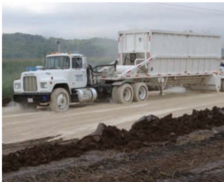
STH 60 near Lodi, Wisconsin: Fly ash is being deposited by special lay-down equipment for mixing with soft subgrade to form a stabilized subbase.
