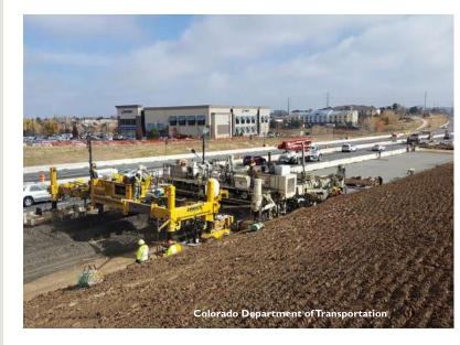
Roughly 1.2 million square yards of fly ash-rich "green concrete" was placed during the construction of 12.5 miles of new express lanes on Colorado State Highway 470.
