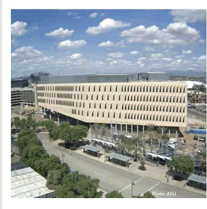
High fly ash mixes were used for structural concrete required to achieve a range of strength requirements for elements including slabs on grade, caissons, decks, walls, and columns. Beyond the concrete mix's strength and sustainability requirements, its use in exposed applications—including stairs, soffits, and flooring—meant it needed to be aesthetically pleasing as well.
