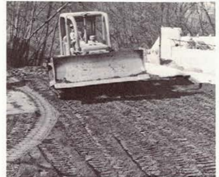
Ash Being Compacted
