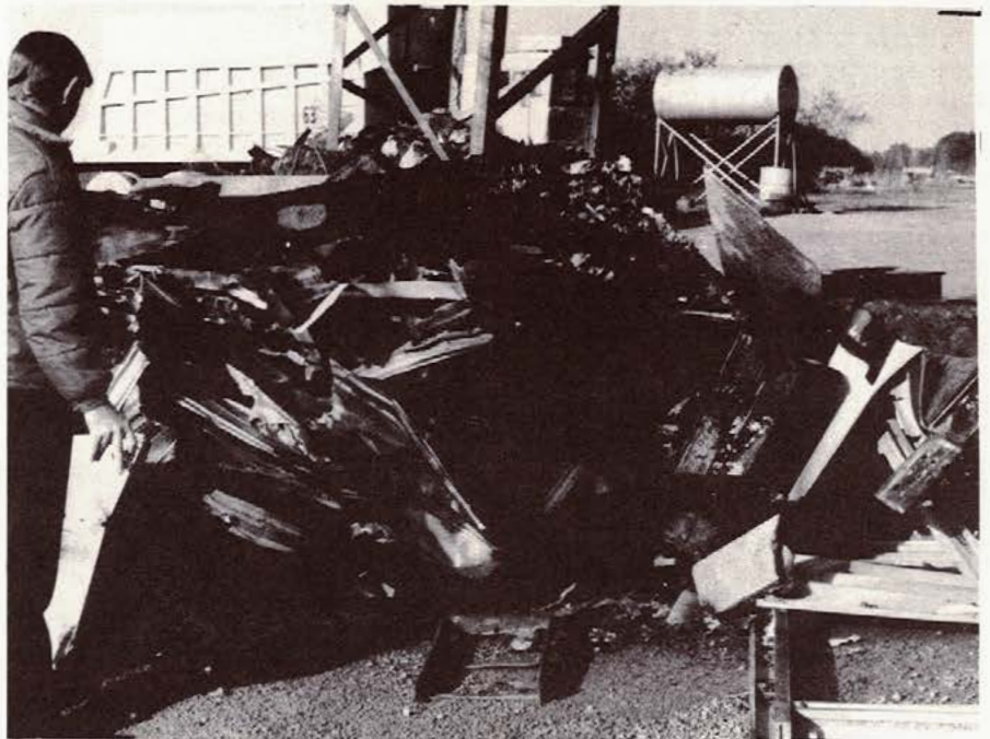
FIRE DESTROYS ASH PLANT —Plant Superintendent Woody Woodall surveys the charred remains of Gifford-Hill's fly ash plant at Cason, Texas. The facility was back in operation within two days. (Photo and story, courtesy Gifford-Hill "TIMES," May 1980)
