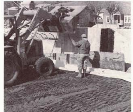
Completed Ash Fill
