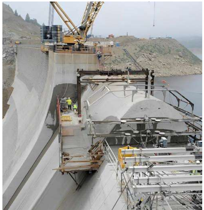
Photo courtesy of Denver Water
