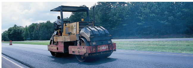
Bottom ash can be used in asphalt paving.
