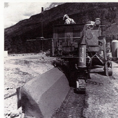
Placing "test" curbs.
