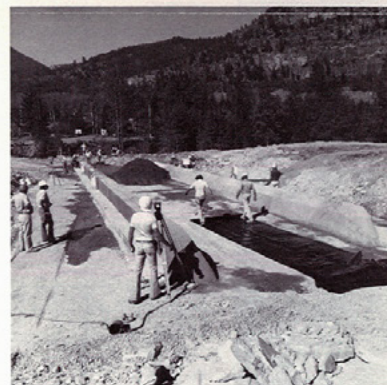
Test strip of RCC concrete.
