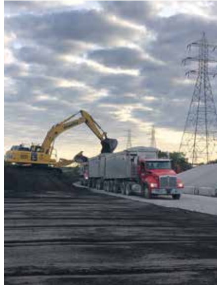
Ash from B.C. Cobb ponds being loaded into railcars and trucks for transport to J.C. Weadock Landfill.
