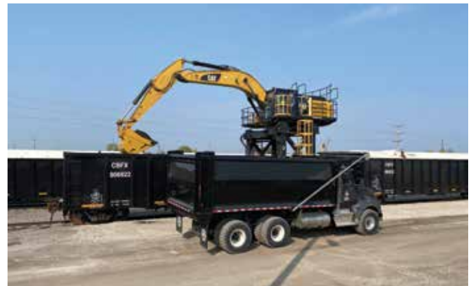
Straddle carrier unloading recycled ash from the railcars at J.C. Weadock Landfill.
