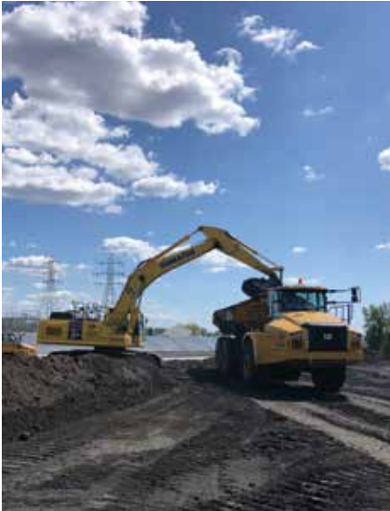
Ash from B.C. Cobb ponds being loaded into railcars and trucks for transport to J.C. Weadock Landfill.
