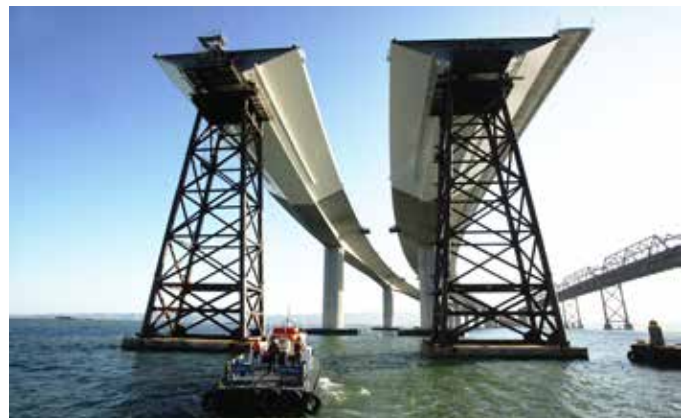
Credit: California Department of Transportation.
