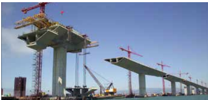
Credit: California Department of Transportation.
