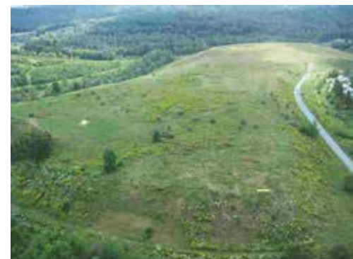
Revloc #1 refuse pile in 2014 after reclamation.
