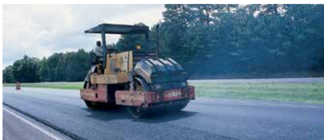
Bottom ash can be used in asphalt paving.
